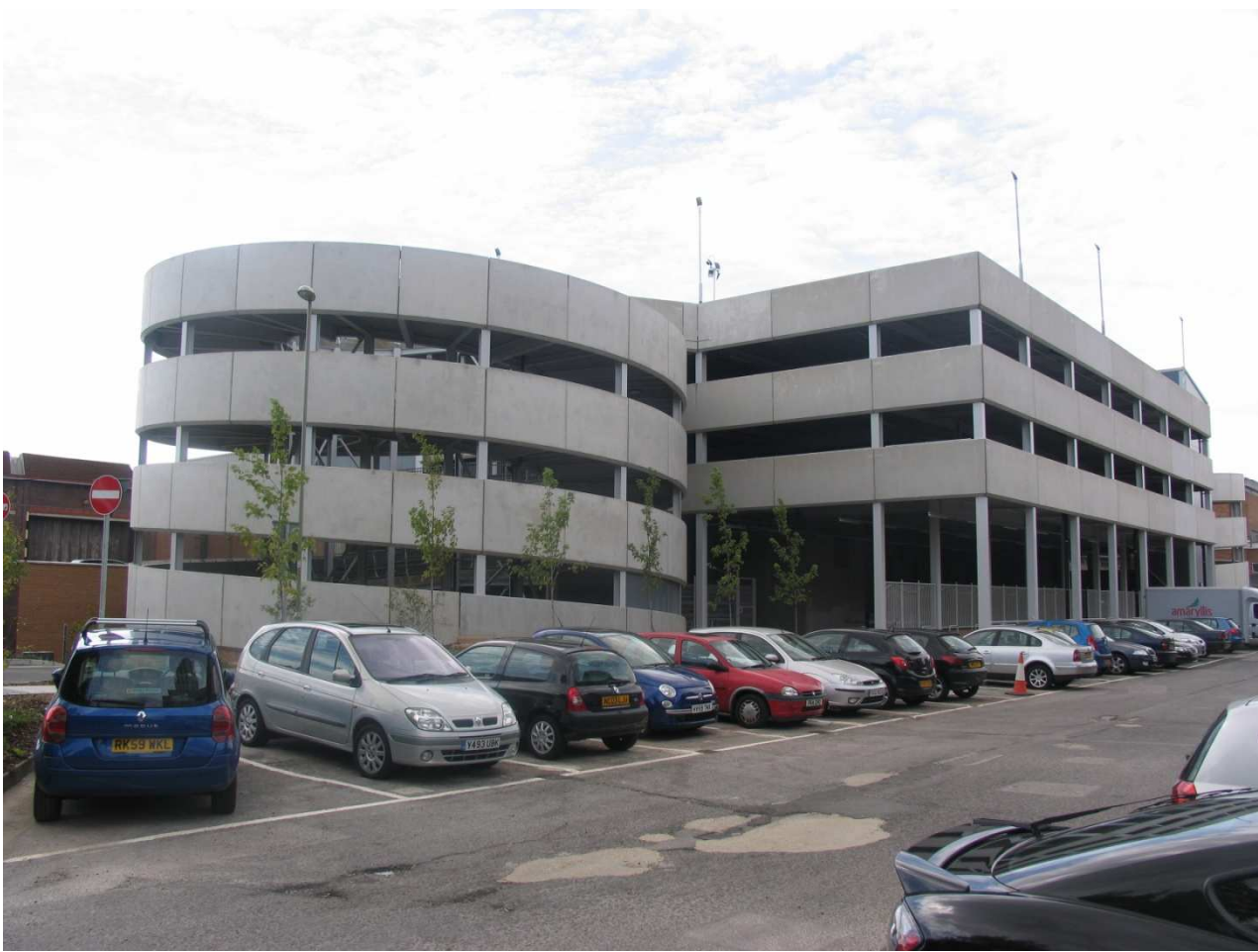
Fareham Shopping Centre Multi Storey car park
